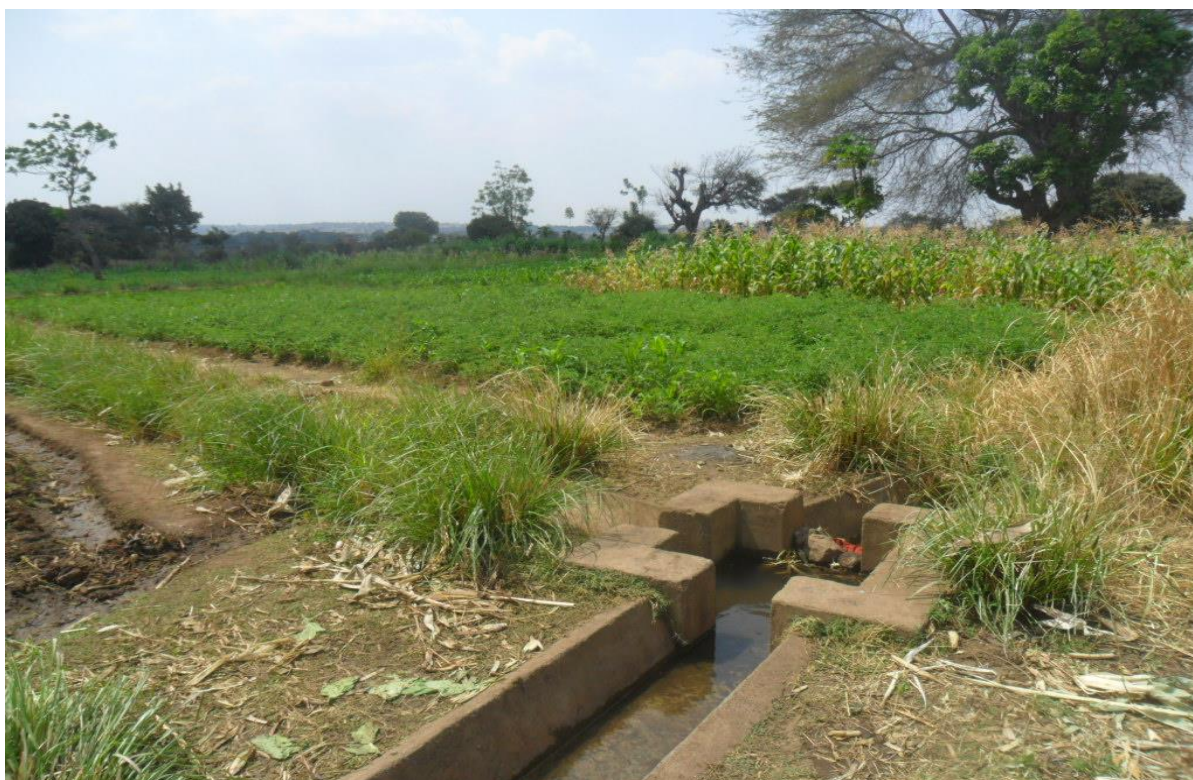
Photo 4.5 Water distribution between adjacent farmer's fields plots one using chameleon on the right-hand side.
